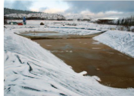
The LDS pond system was converted to the HDS process.
