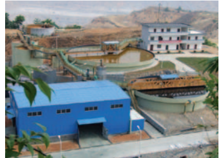
The Dexing plant recovers a high grade copper product that is sold to offset water treatment costs; the treated water is re-used at the site.
